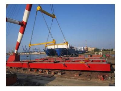
Fig. 7. The two segments of the steel deck over the pylons
